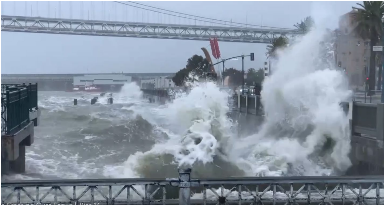
Figure 6. Wave overtopping for existing conditions, March 2023.
